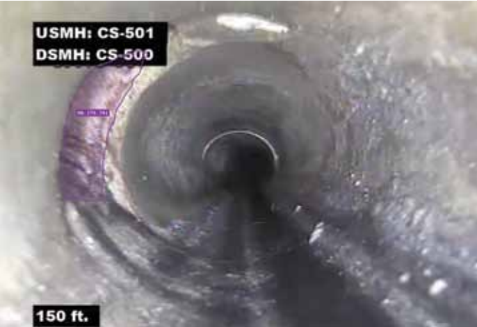
Figure 5. Screenshot from an updated video inspection file following an AI scan. The purple overlay depicts Tap Break-in/ Hammer (TB) with an AI confidence interval of 79.7 percent.
