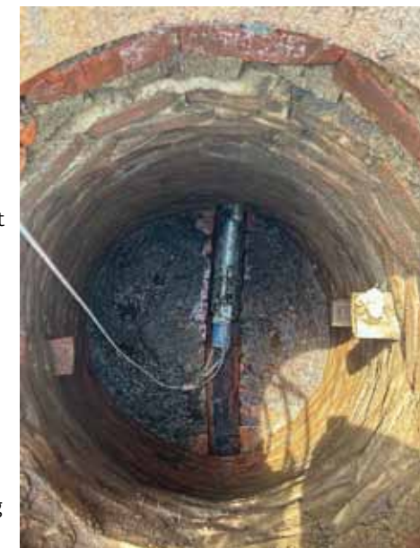
Figure 2. CCTV inspections involve operating a robotic crawler mounted with a camera through the gravity sewer following the standards set forth by the PACP
