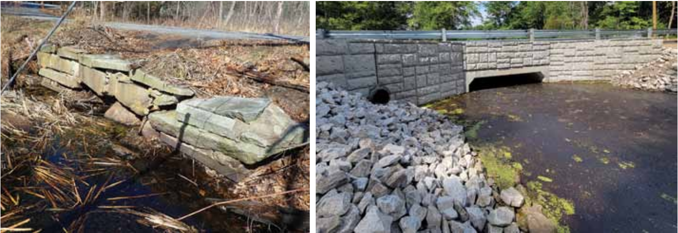
Pond Brook culvert, pre-construction (April 2022) and post-construction (August 2024)
