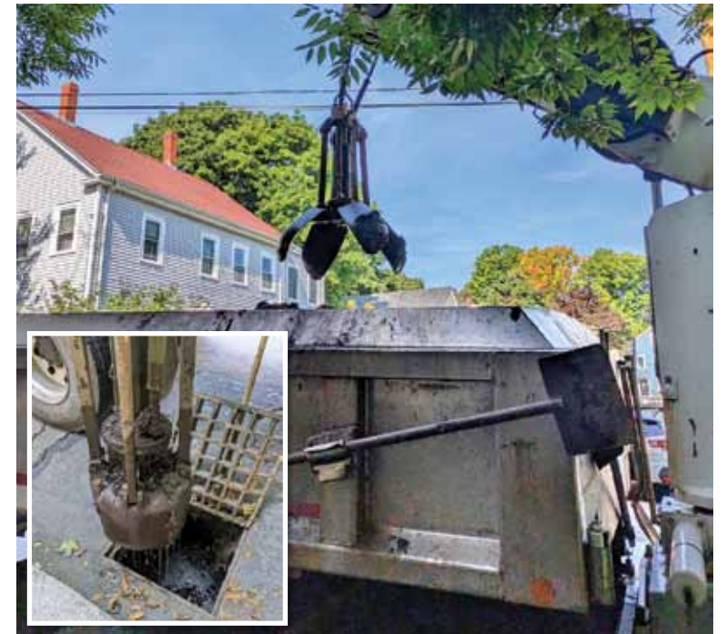
Catch basin cleaning
