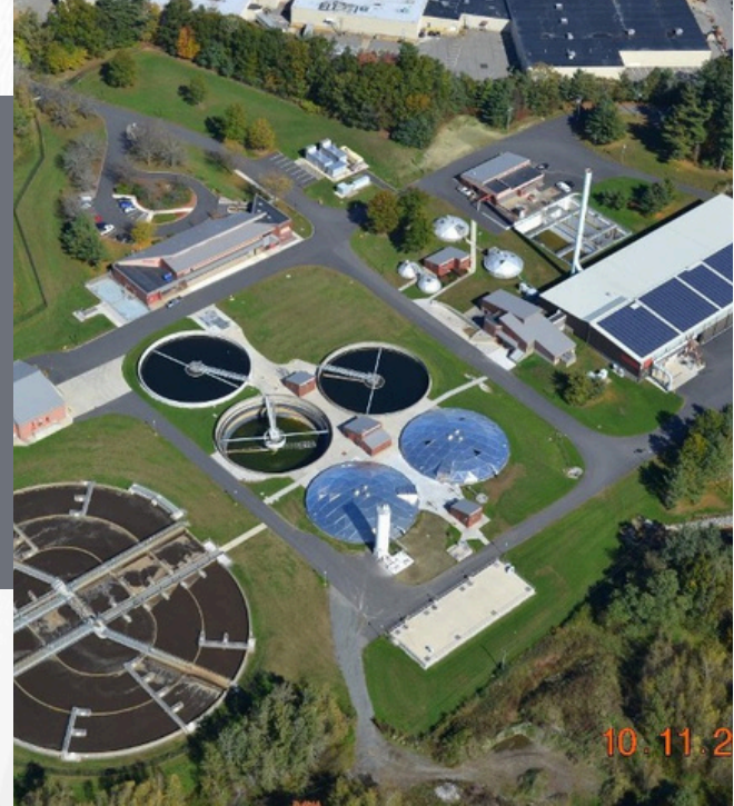
Westborough, MA WWTP
