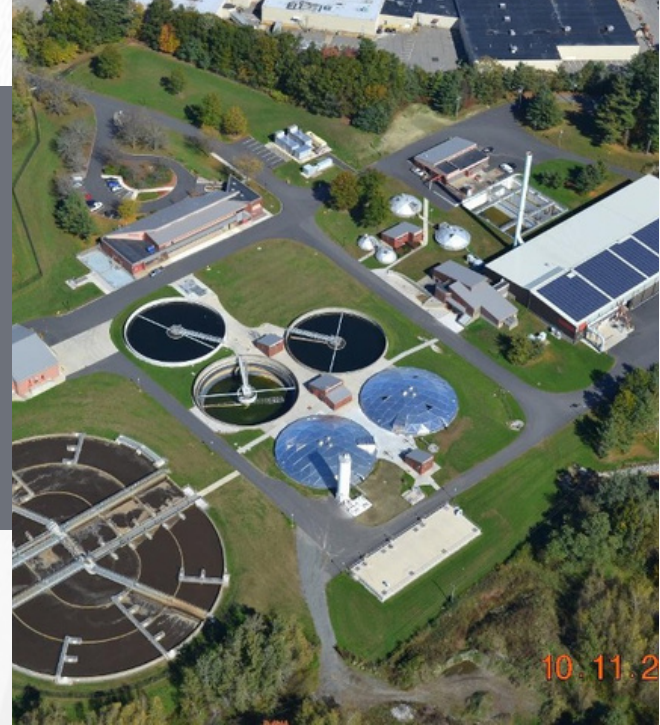
Westborough, MA WWTP
