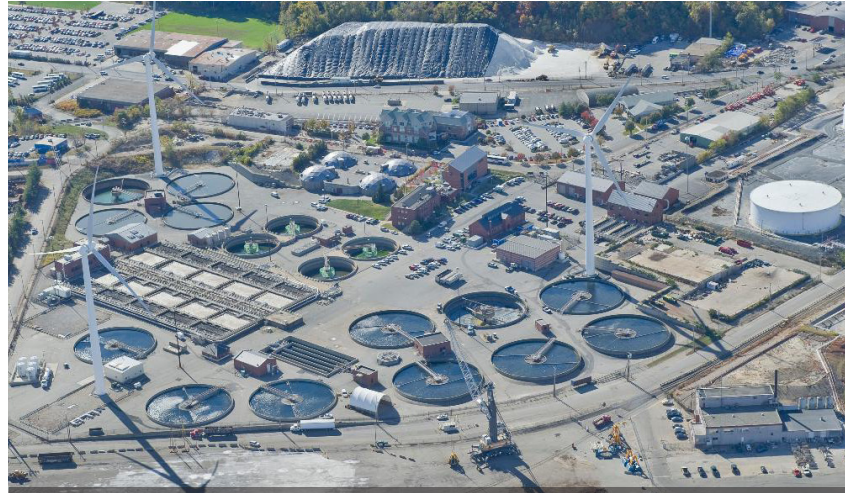
Field's Point Wastewater Treatment Facility, Narragansett Bay Commission
