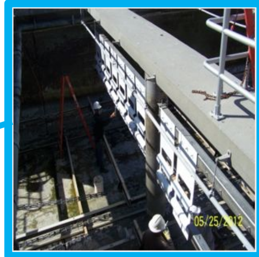
Flocculation Baffles
