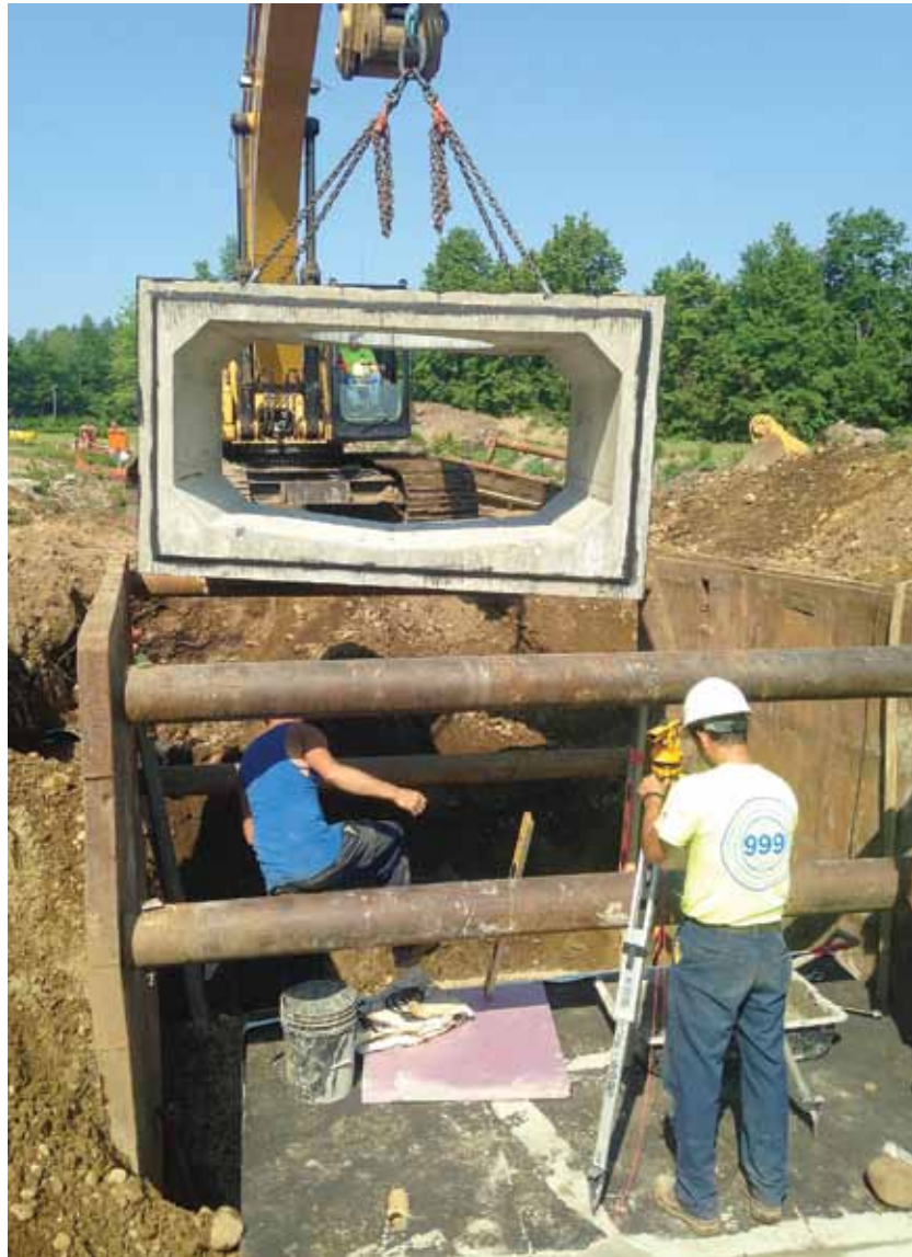
Figure 5. Trench box support in use during construction
