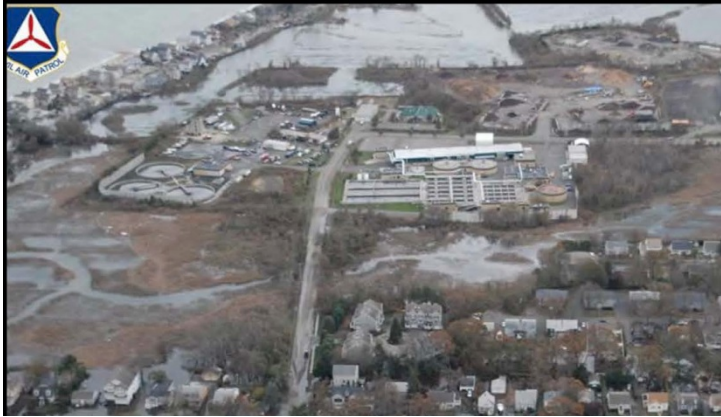
Fairfield WWTP (US Coast Guard)
