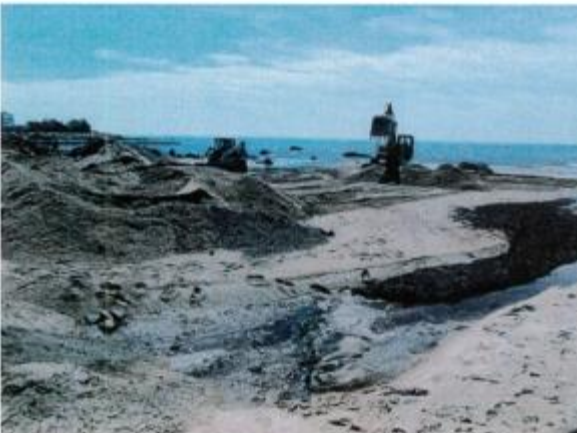
Exposure of Water Main and replacement of the Sand
