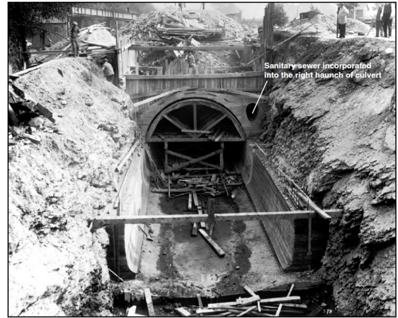
Figure 11. The culverting of Stony Brook at Forest Hills, about 1905.
