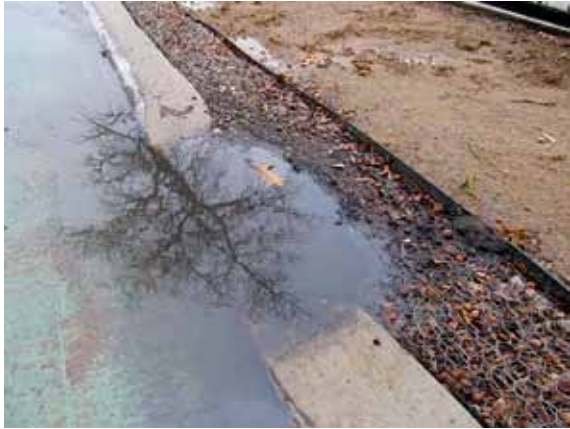
Excess sediment buildup preventing runoff from entering (an unplanted) ROWB
