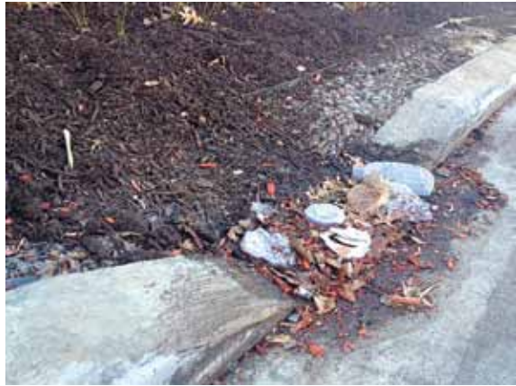
Stone and improper grading preventing runoff from entering the ROWB
