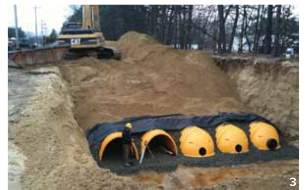
1. Expansion of the upper Granby Road detention and infiltration basin (during construction) 2. Expansion of the upper Granby Road detention and infiltration basin (post-construction) 3. Construction of the Champion Drive infiltration system
