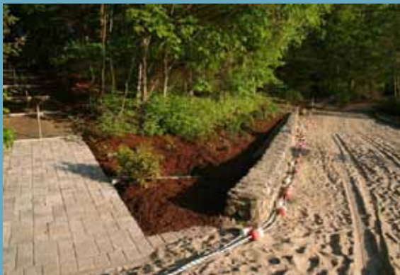
Sherborn Farm Pond, Sherborn, MA – Permeable Pavers, Rain Garden and Groundwater Recharge
