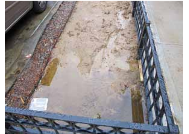
Ponding water shows poor infiltration, likely due to compacted engineered soil
