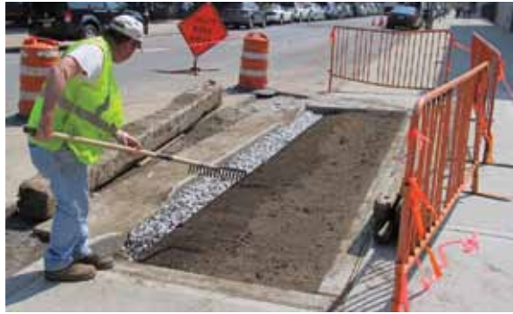
Pedestrian barriers used as ROWB protection during construction
