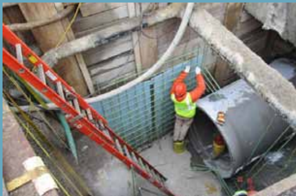
Reserved Channel Sewer Separation Project, Boston, MA – Construction of New Drain Manhole
