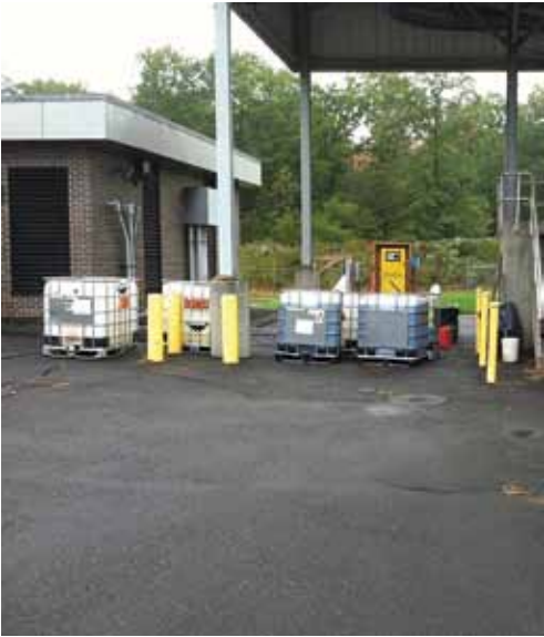
Figure 4. Ferric chloride totes at grit chamber
