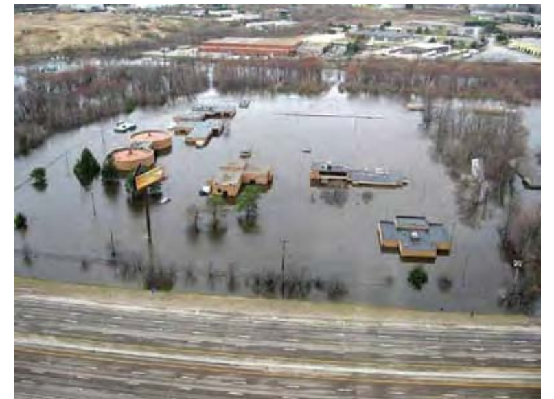
The flooding of the Warwick WWTF on March 30, 2010, resulted in $15 million in damages
