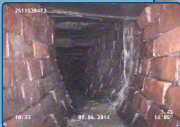
Evaluation of Brick Sewer with Slate Roof, Boston, MA
