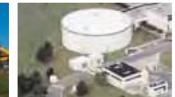
Storm Water Equalization Tank
