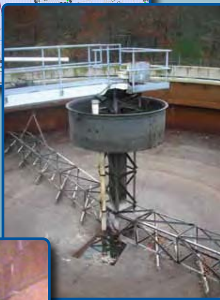
Conditions Survey at Water Pollution Control Facility, Dartmouth, MA
