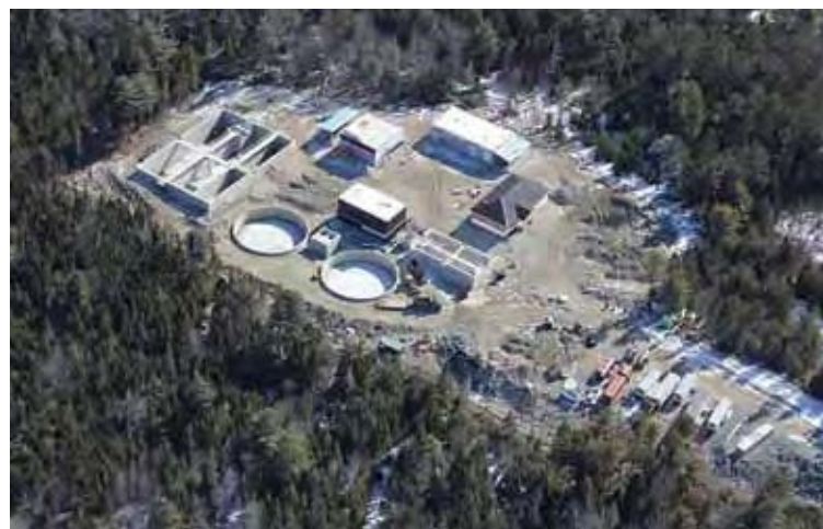
Ellsworth, Maine WWTF under construction
