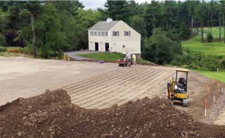
Figure 4. Drip dispersal system under construction at Quail Ridge in Acton, Mass.
