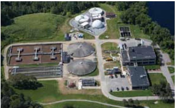
Figure 5. Pre-construction and post-construction
