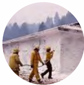
Firefighting Foam (AFFF)
