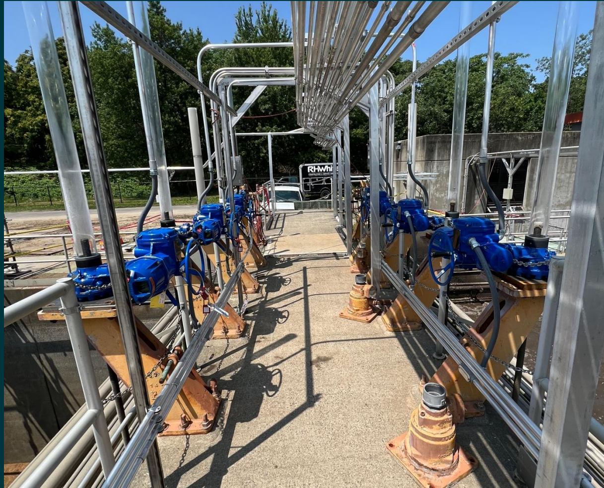
Slide Gate Actuators – 4 per Basin to Control Flow
