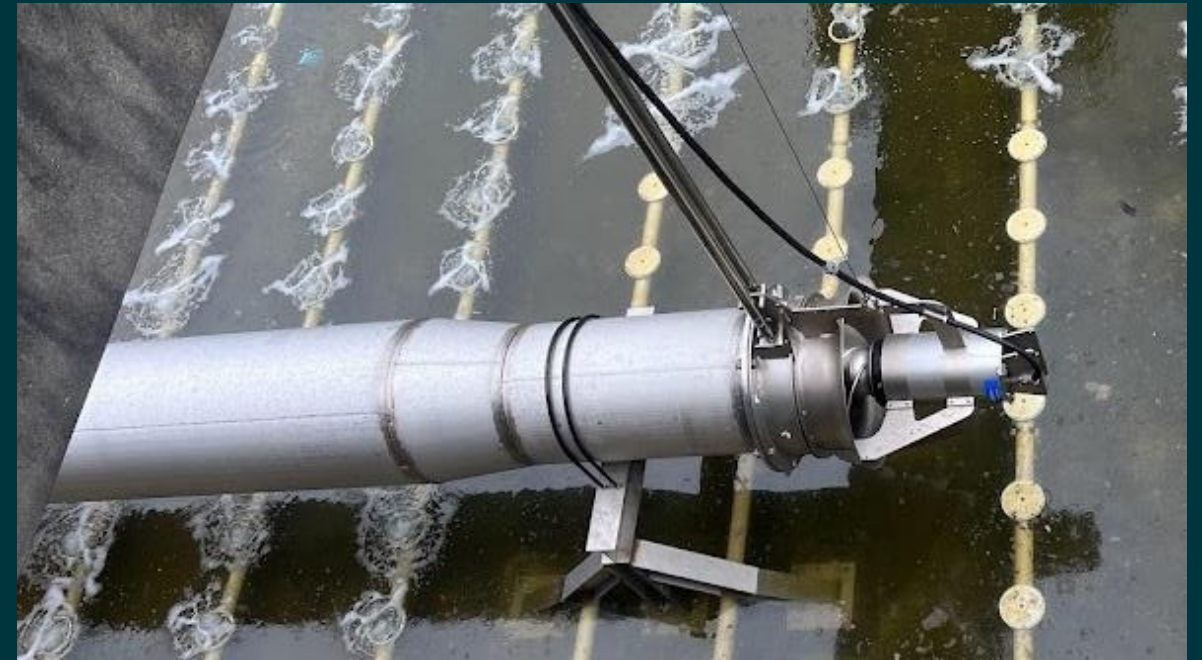
40 HP Axial Flow MLR Pump
