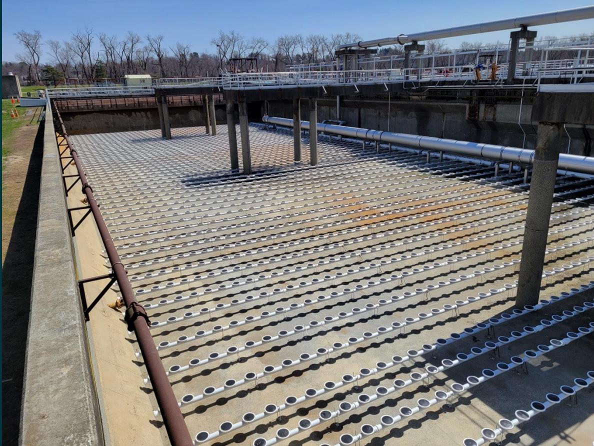
Aeration Diffusers –6496 per Basin Across 9 Grids
