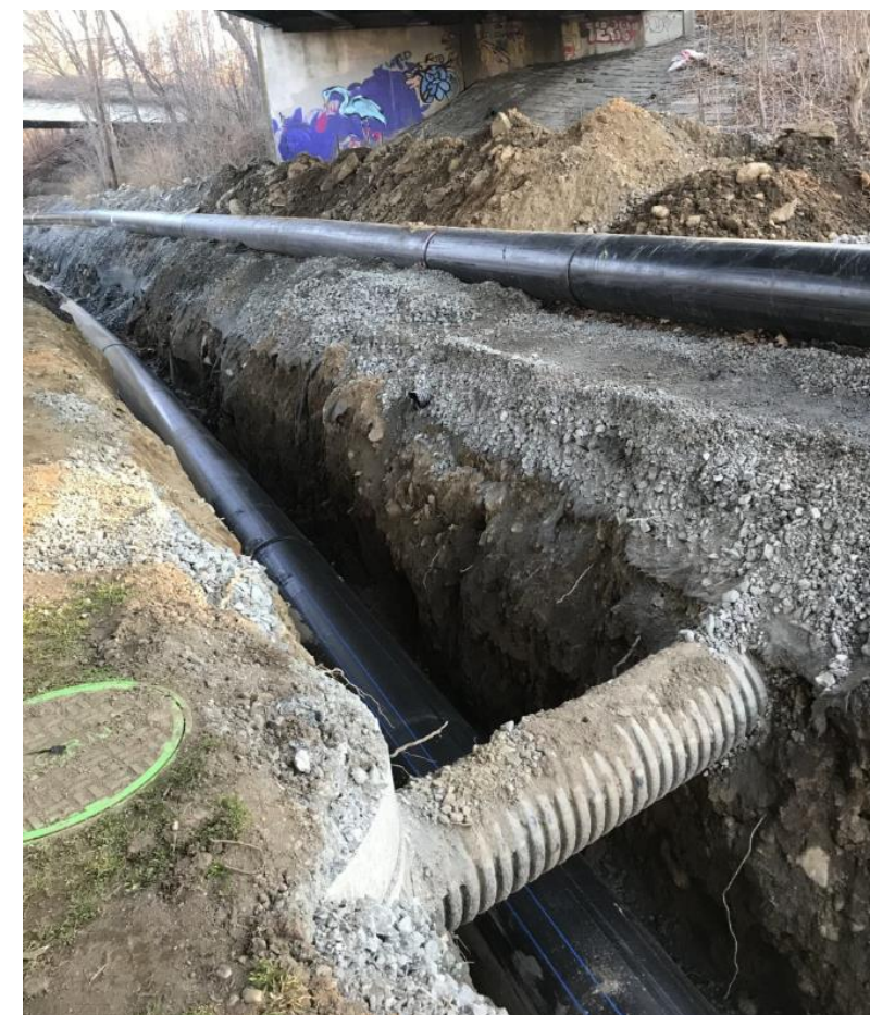
HDPE Pipe Installation – navigating existing infrastructure
