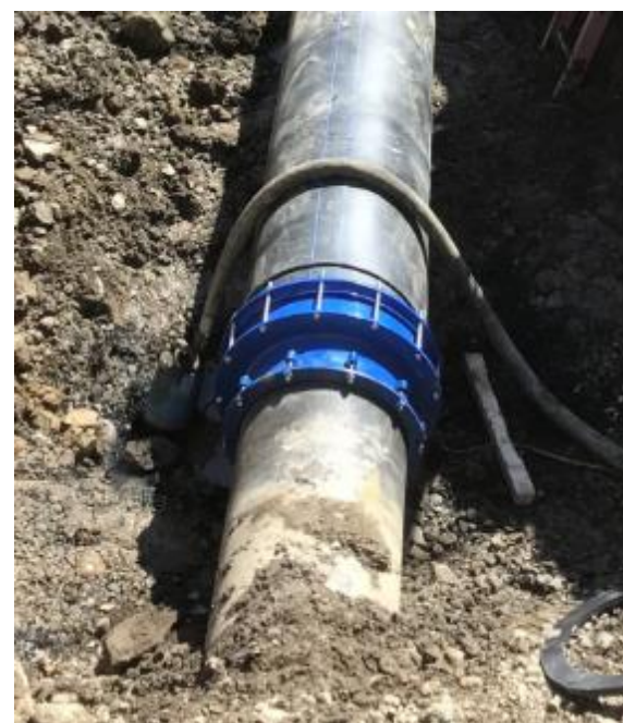
HDPE – DIP coupling
