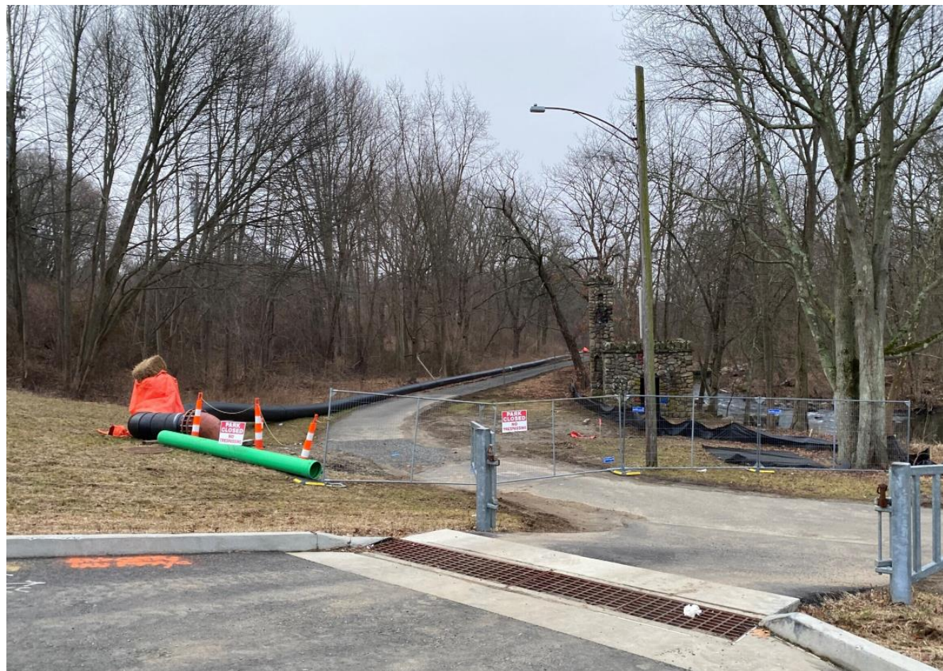
Upstream connection for temporary bypass
