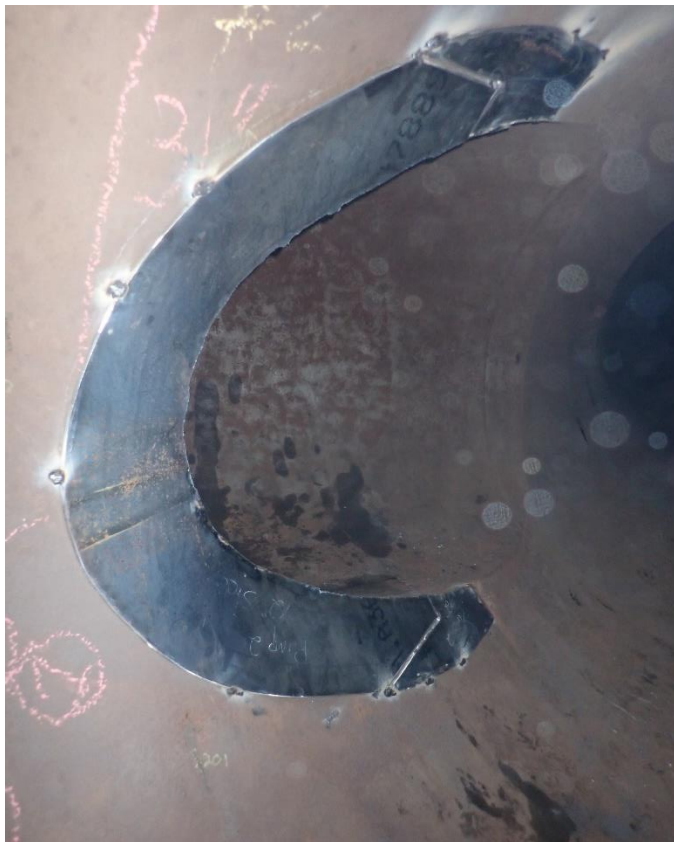
Weld repairs: Discharge crotches
