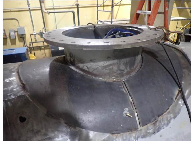
Manhole Installation
