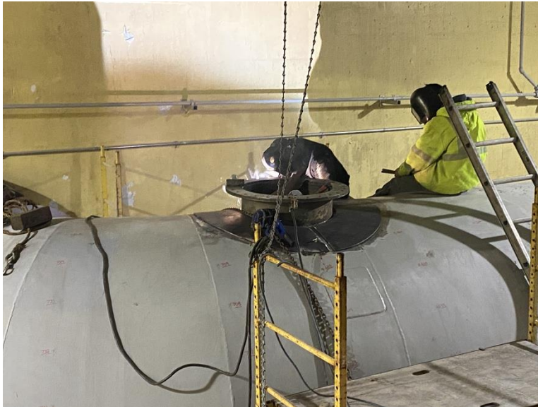
Manhole Installation
