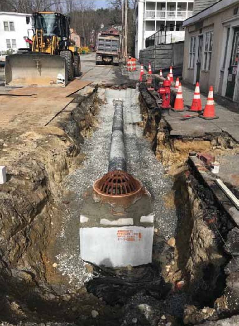
Construction of green infrastructure during the CSO 010 project, in this case a bioretention cell
