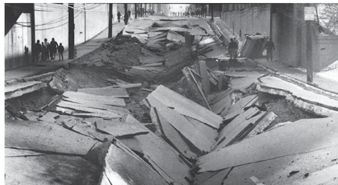
in 1981, a sewer exploded in Louisville, Kentucky—caused by a hexane leak into the sewer from a soybean processing plant
