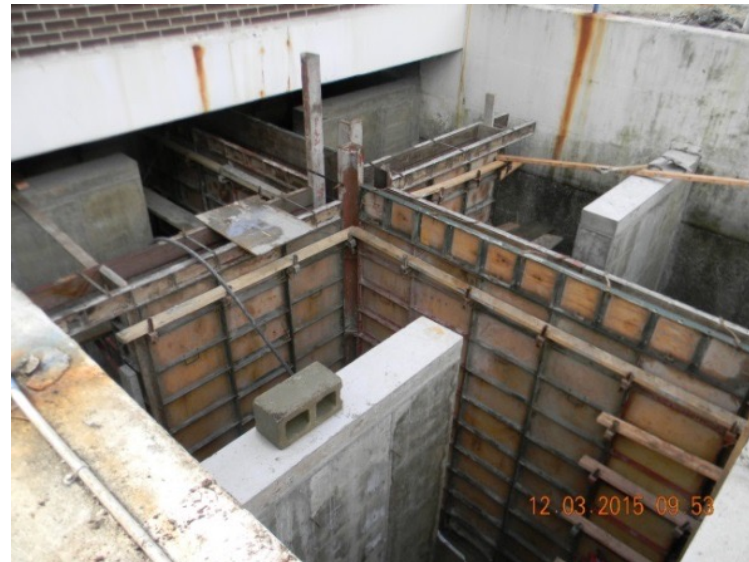
Rehab Chlorine Contact Tank
