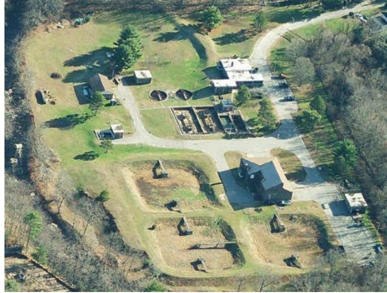
North Plant – Design Flow = 1.09 MGD
