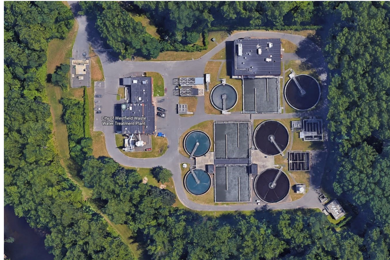
Source: City of Westfield Water Recovery Facility, October 2023.
