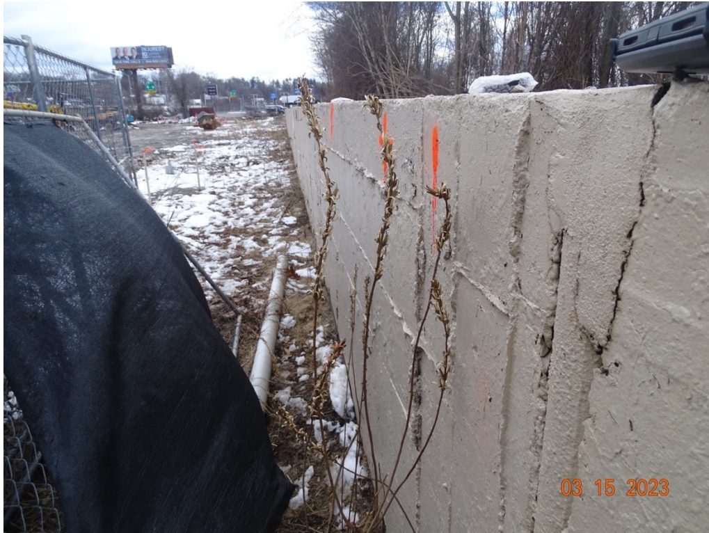
Army Corps Flood Wall – View from North to South SRA Property
