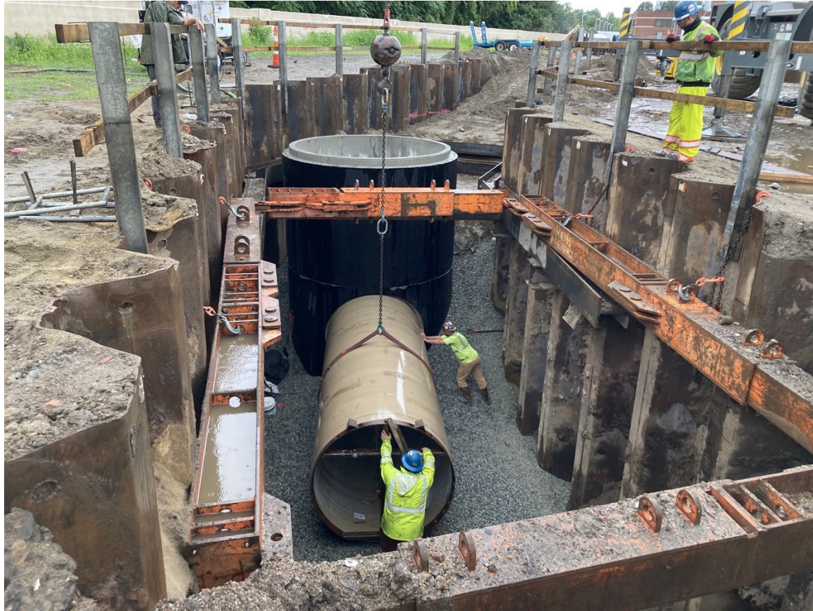
MIS Transfer Pipeline Installation – 72-Inch Pipeline and 10-Foot Manhole SRA Property
