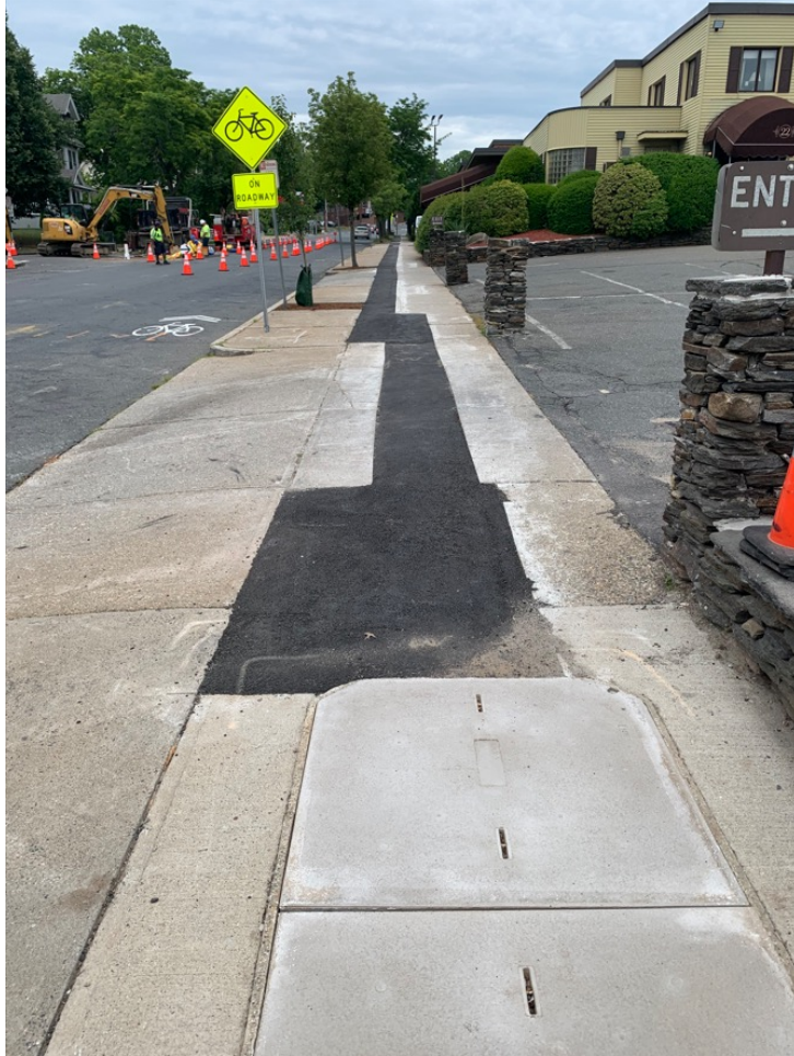
CATV Duct Bank Relocation to Sidewalk Locust Street
