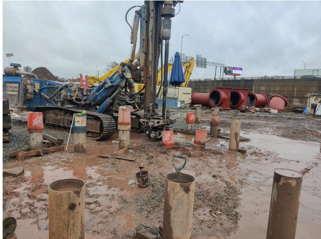
Drilled Micropile Installation for MIS Diversion Foundations SRA Property
