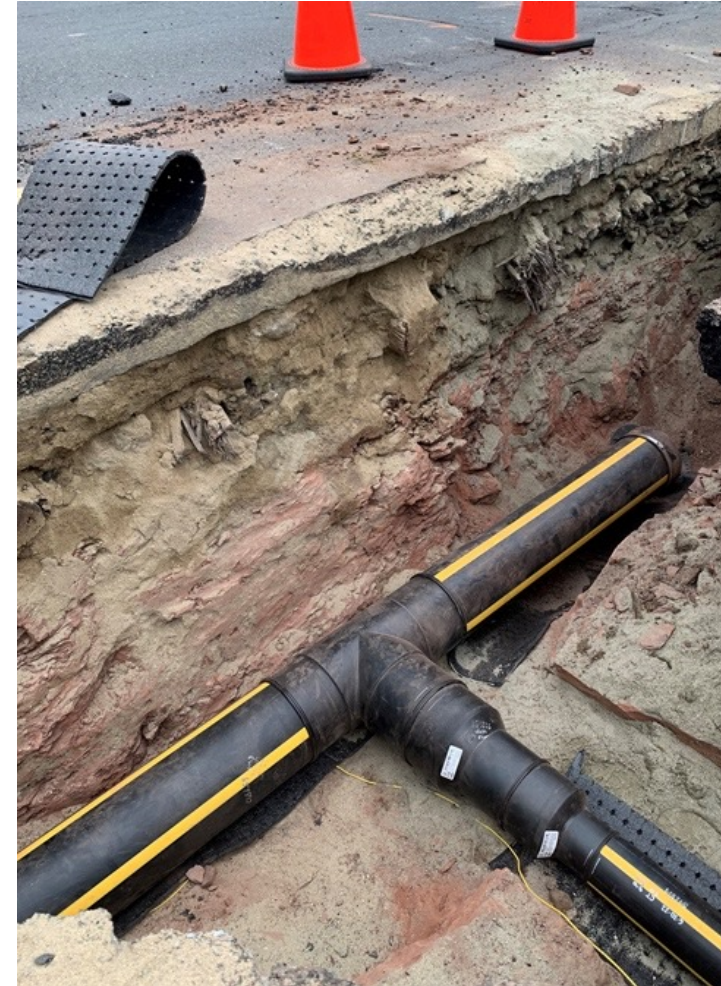
8-Inch Gas Main Replacement – Ledge and Rail Ties Locust Street
