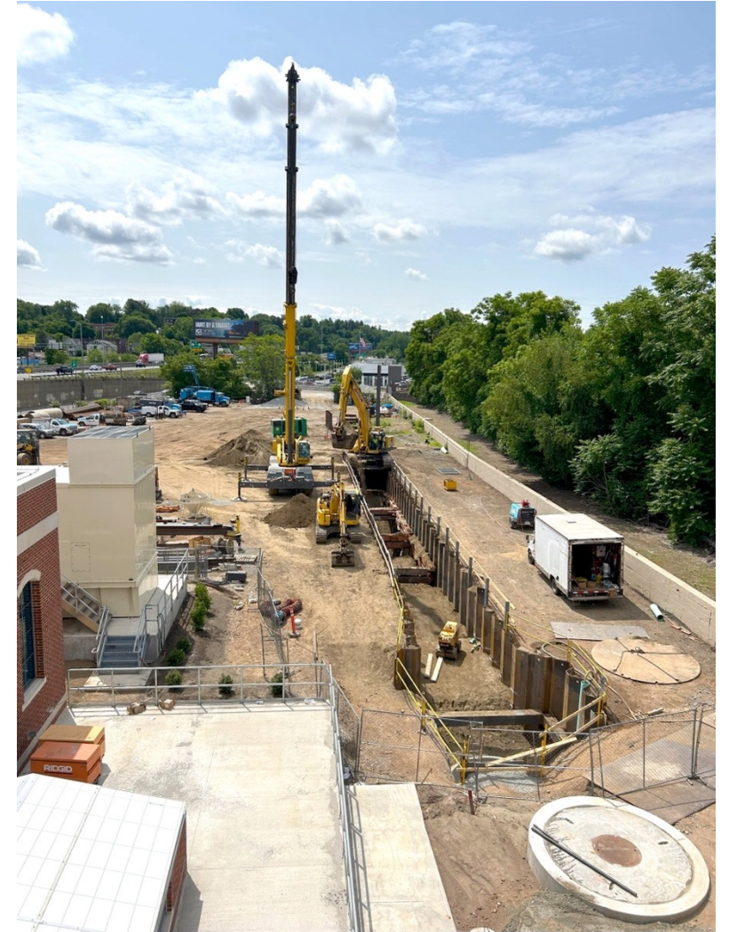
MIS Transfer Pipe Installation – View from York Street Pump Station
