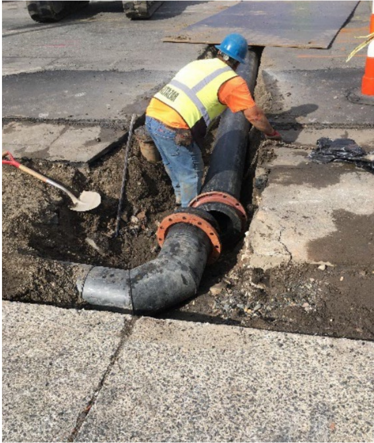
Temporary Sewer Bypass Piping Locust Street and Main Street
