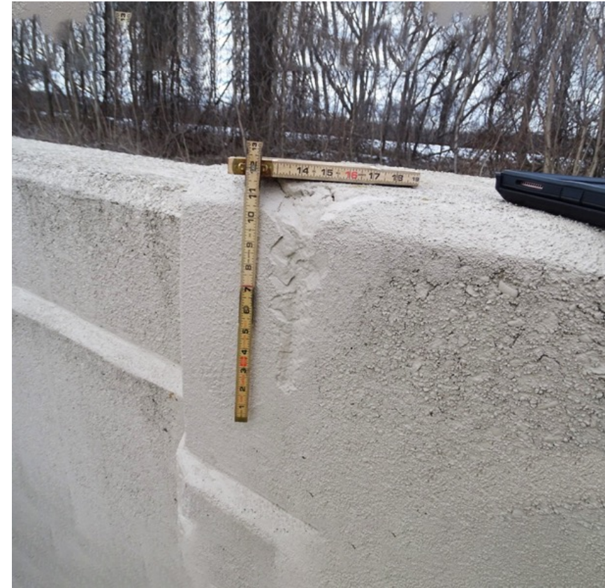
Required Careful Pre-Construction Survey and Monitoring During Construction SRA Property
