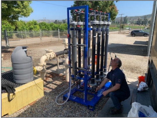
PFOA Treatment - Lead Vessel
