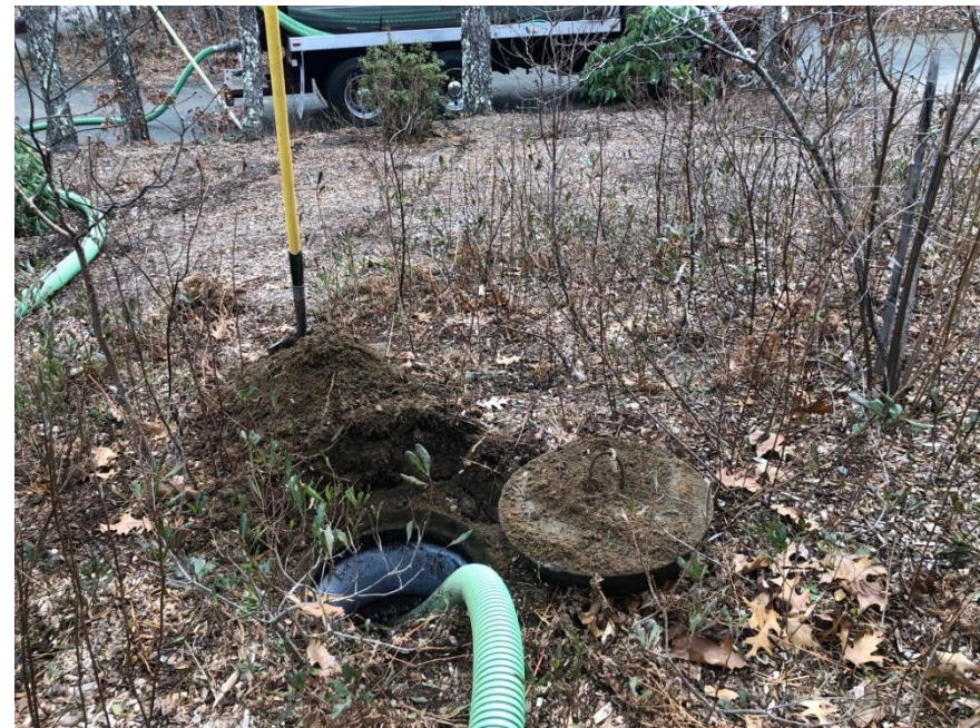
Septic Tank being pumped out
