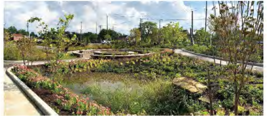
Figure 3-41. Rain Gardens/Vegetated Bioretention Areas
