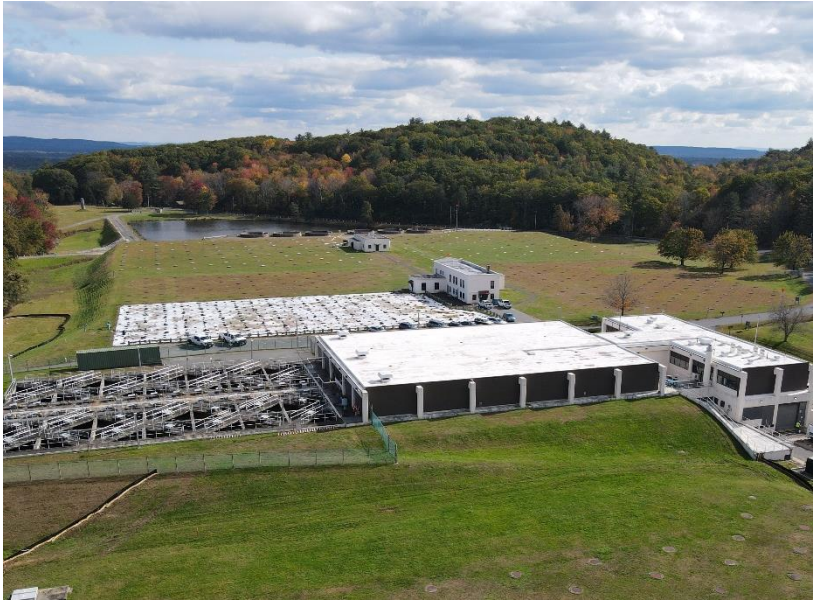
West Parish Filters Water Treatment Plant, Westfield MA
