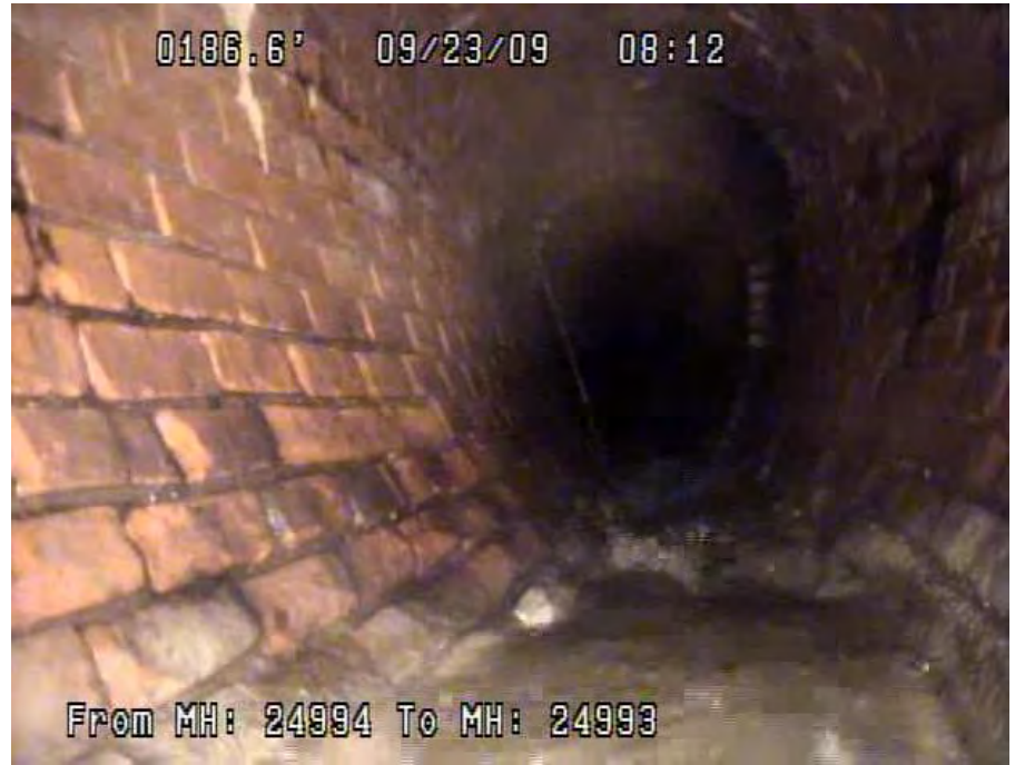
Missing Mortar
