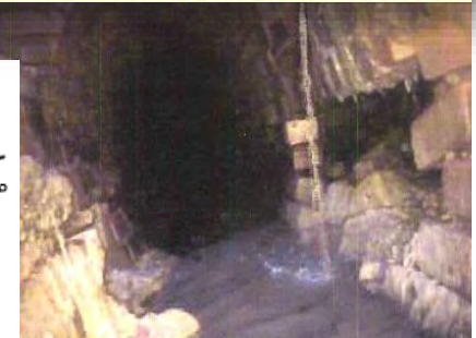
TWENTY-SIX FOOT ROCK EXCAVATION FOR SIX-FOOT CEMENT SEWER
