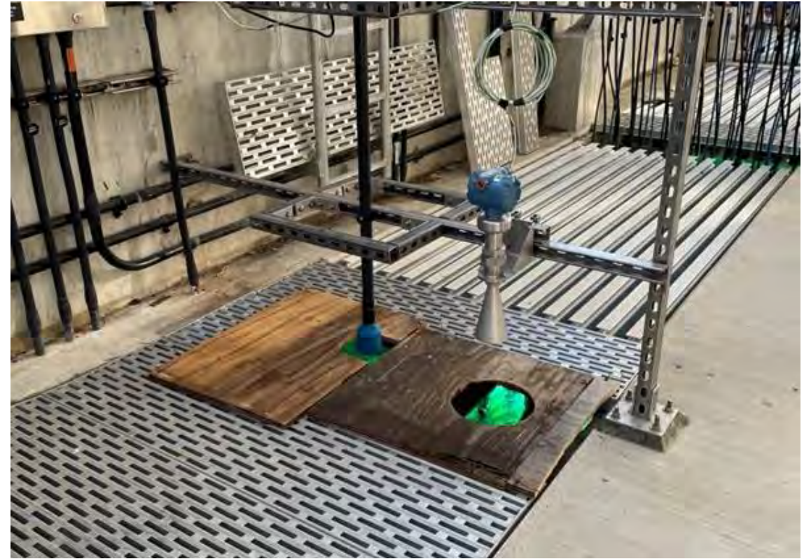
Compare channel water depth to effluent weir gate position
