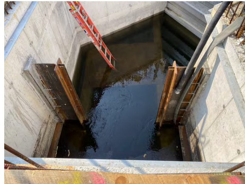
Temporary Bulkhead In Place
