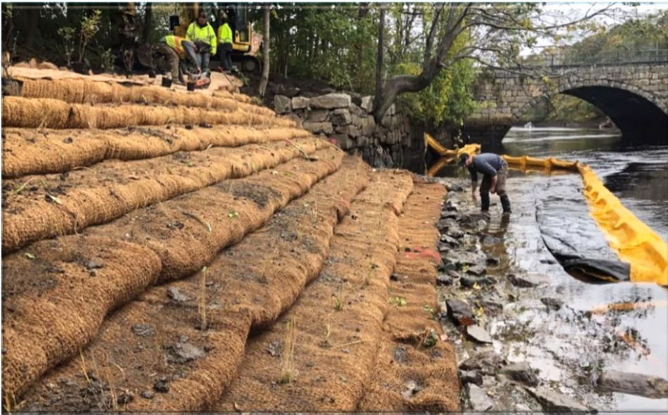
FESL with Toe Rock Upper Bank Failure Treatment
