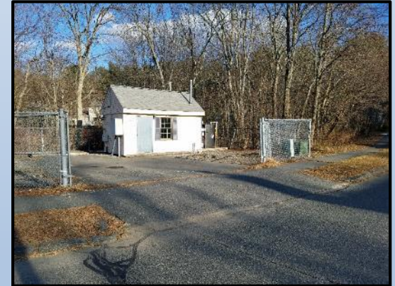
Arrowwood Pump Station
