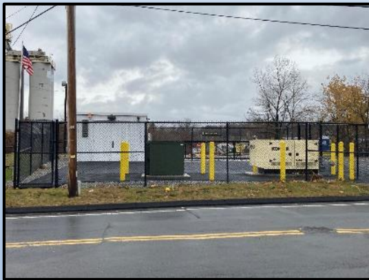
BT Pump Station
