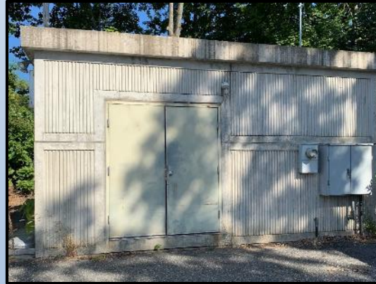
Edgemere Pump Station
