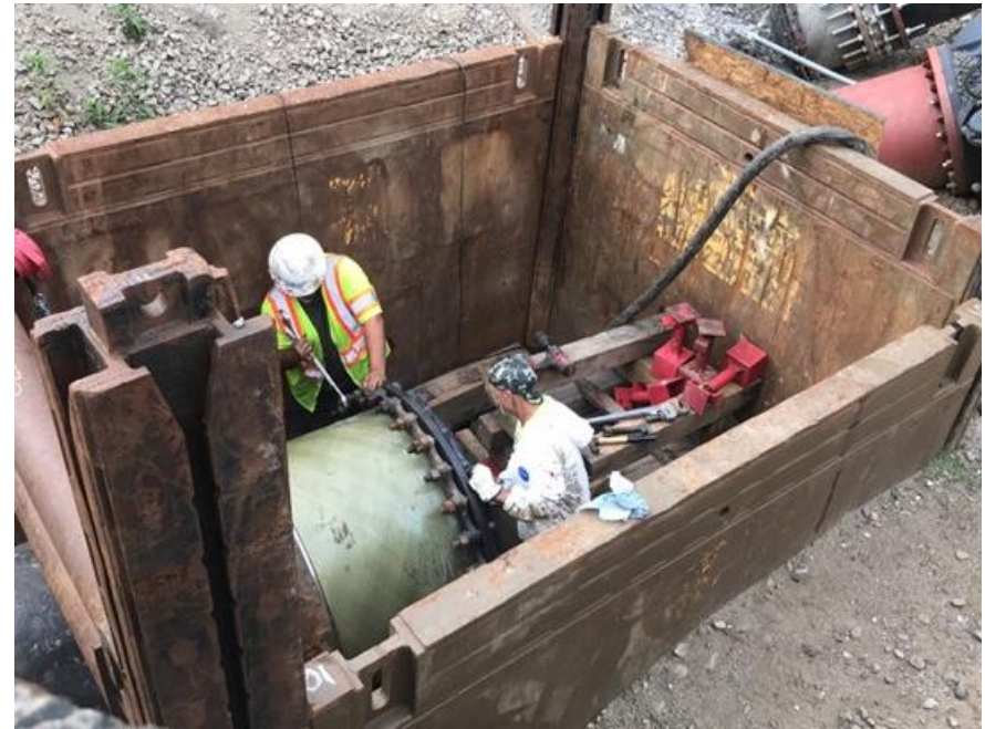
Pressure testing liner
