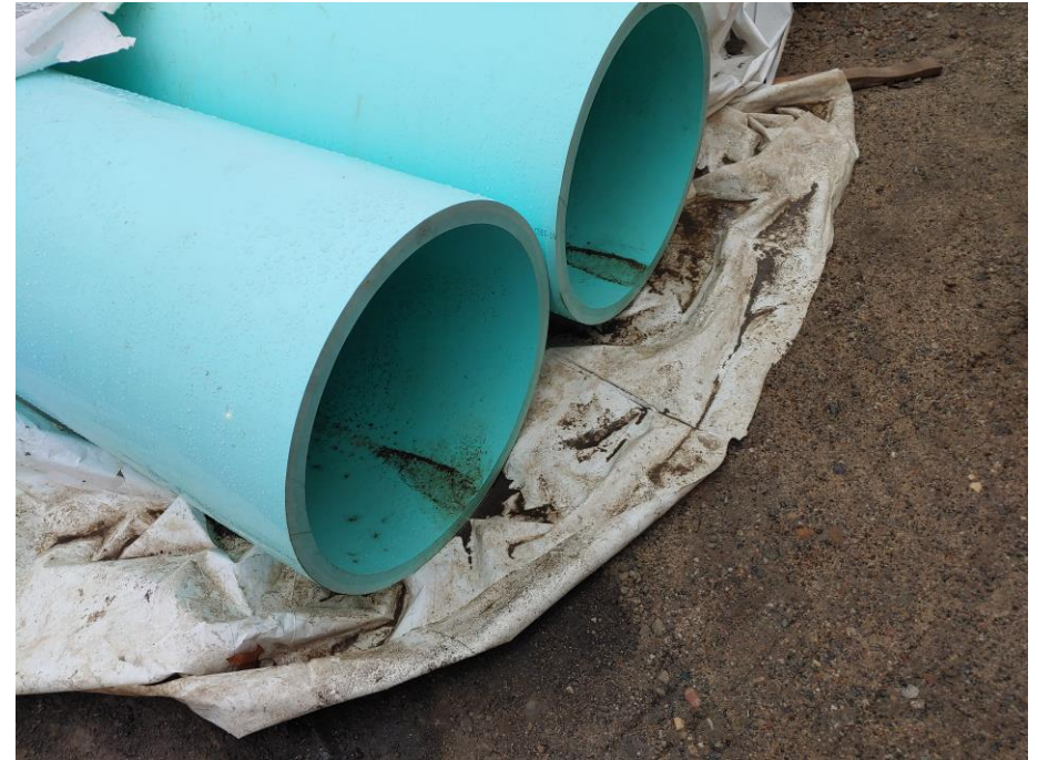
20" Fusible PVC Slipliner
