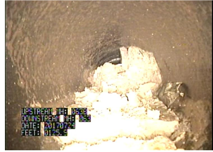
Collapsed Pipe
