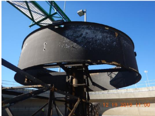
Intermediate Clarifier – Internals – Peeling of the topcoat was typical throughout Intermediate Units exposing a white colored undercoat/product.
