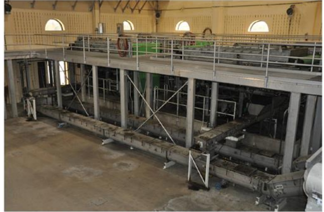
Belt Presses, Cross Conveyors, and Transfer Conveyors
