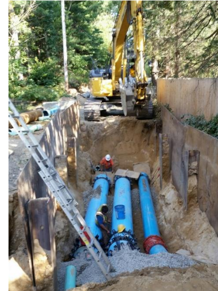
PVC Force Main Installation
