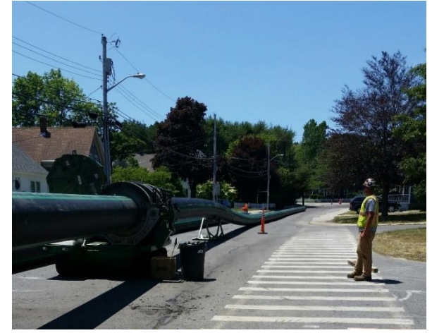
HDPE Force Main For Slip-Lining
