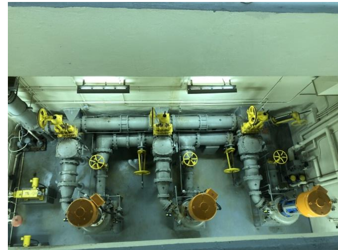
Site Visit to Pump Station
