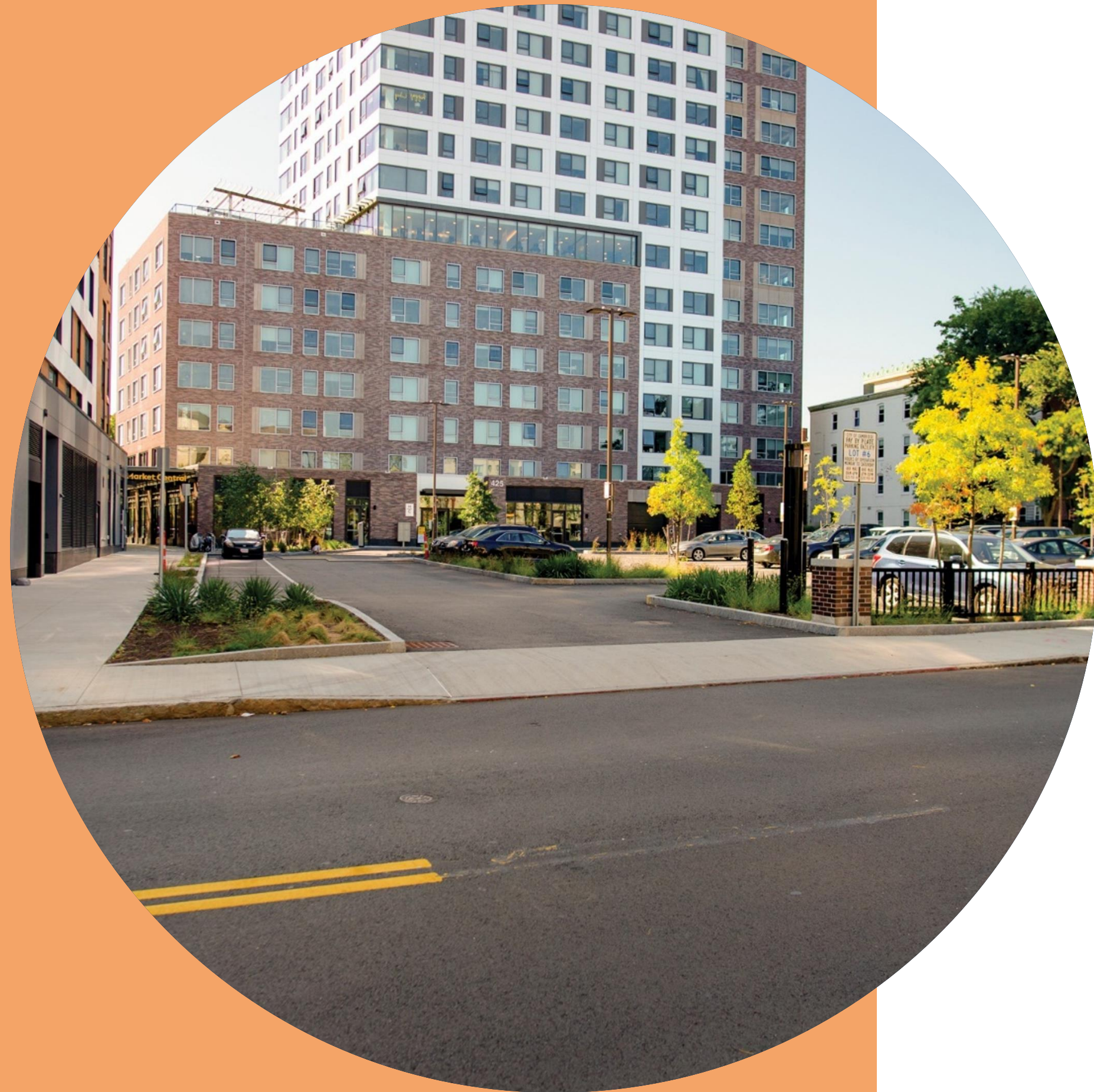
Completed Parking Lot No. 6 Stormwater Tank
