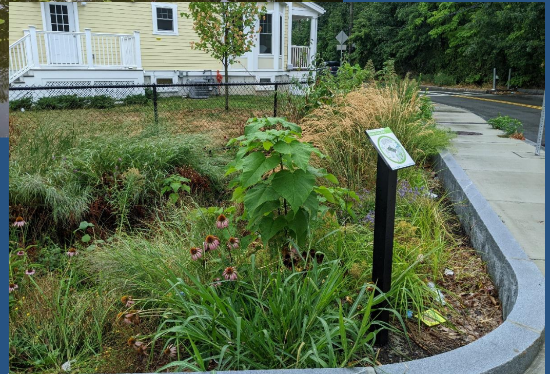
Bioretention Planters and Educational Signage at New England Avenue, Boston
