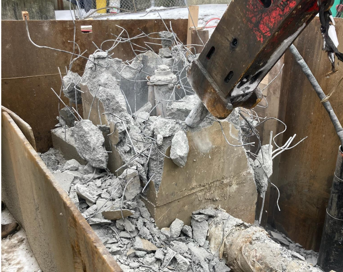
Large concrete thrust blocks discovered in field
