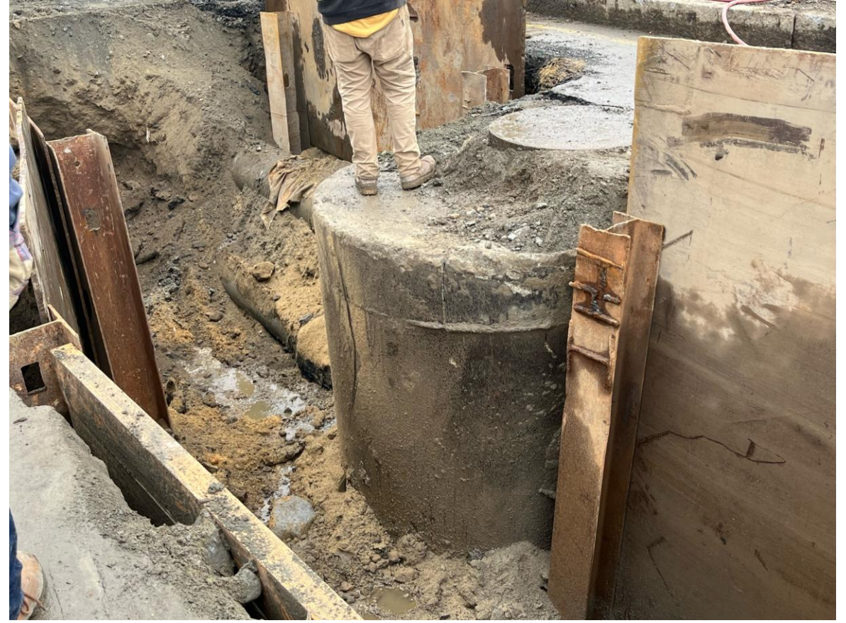
A Swampscott manhole installed on top of Nahant's force main
