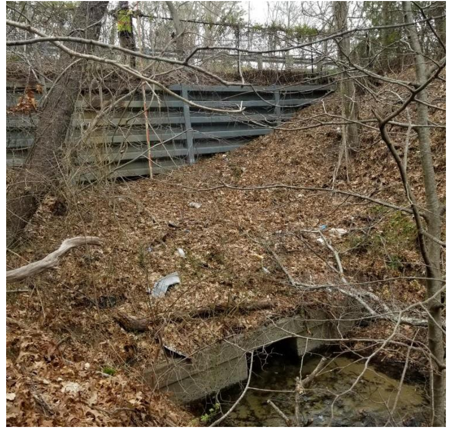
Falmouth Road (Route 28)
