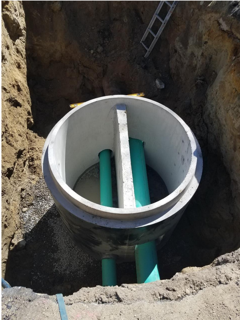
Dual Access Manhole
