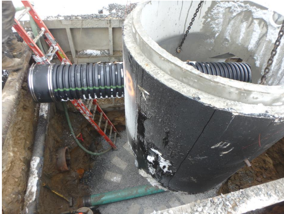
Doghouse manhole over existing sewer
