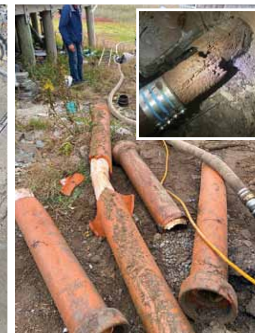
Figure 12. Existing sewer service found with damaged liner and (inset) in broken condition
