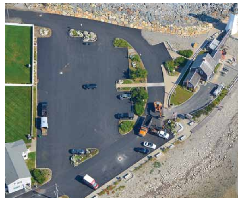
Figure 11. Final surface restoration near lighthouse
