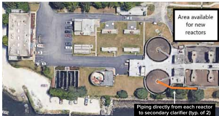
Figure 3. WWTF prior to upgrade
