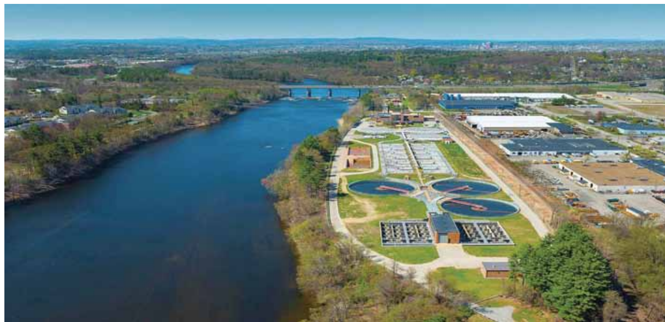
Manchester, New Hampshire WWTP
