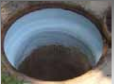
FLEX SEAL UTILITY SEALANT® An aromatic urethane noted for extreme toughness, elongation, abrasion resistance, and longevity.
