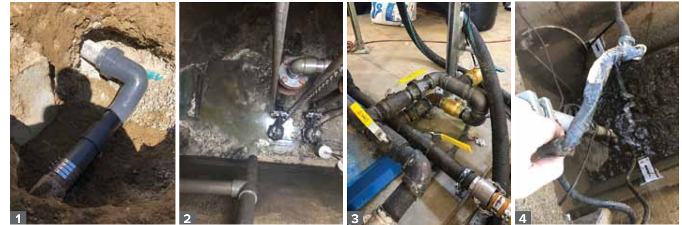
1. Repaired aeration line 2. Overdosing sodium bicarbonate resulted in blockages and precipitation in feed lines 3. Improper materials used on heated line 4. Temporary spliced wiring job that becomes long-term
