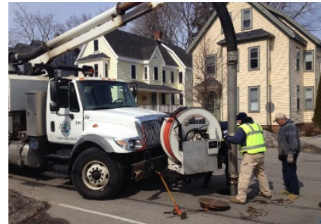
Catch Basin Cleaning
