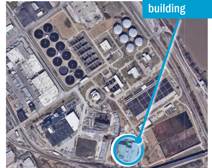
Bissell Point WWTF
