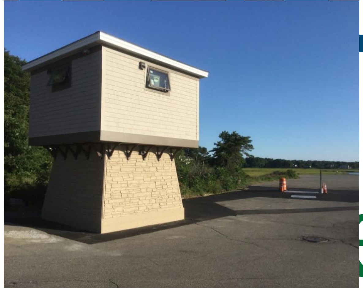
Ogunquit Pump Station No. 1 (after upgrade)
