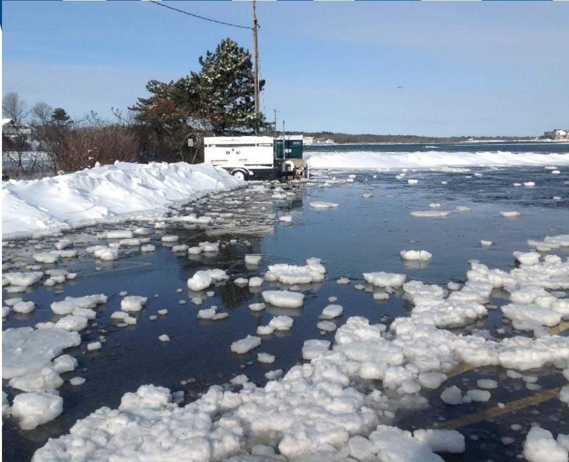
Ogunquit Pump Station No. 1 (before upgrade)
