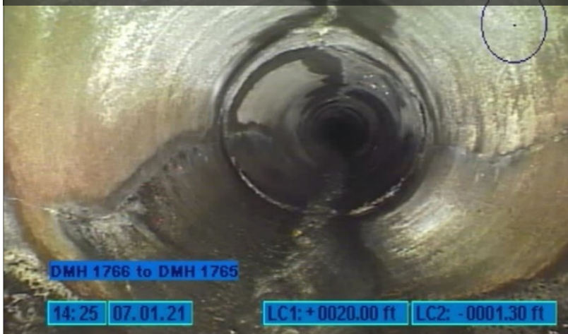
Pipe with cracks
