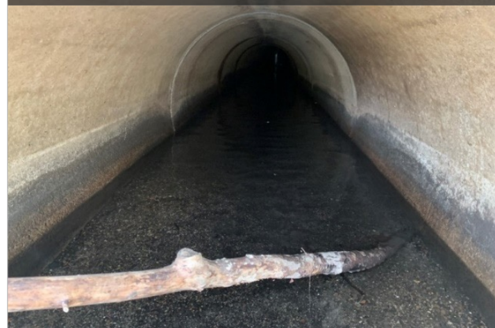
Pipe 1/3 full of sediment
