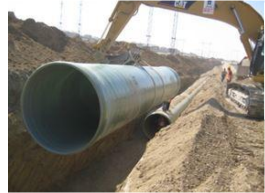
Storage and Flow Diversion Example: Large Diameter Pipe Installation
