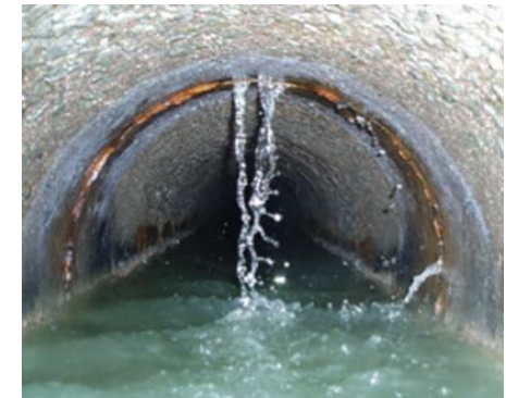
Reduce Pipe Infiltration
