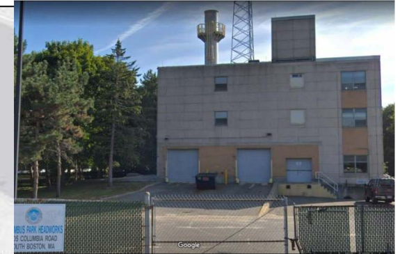
Columbus Park Headworks Facility (MWRA)
