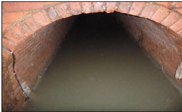
Dorchester Interceptor 54" Circular Brick Pipe
