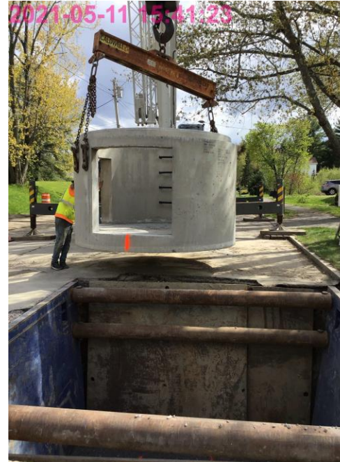
Brighton Avenue Sewer Separation Manhole Installation Summer of 2021
