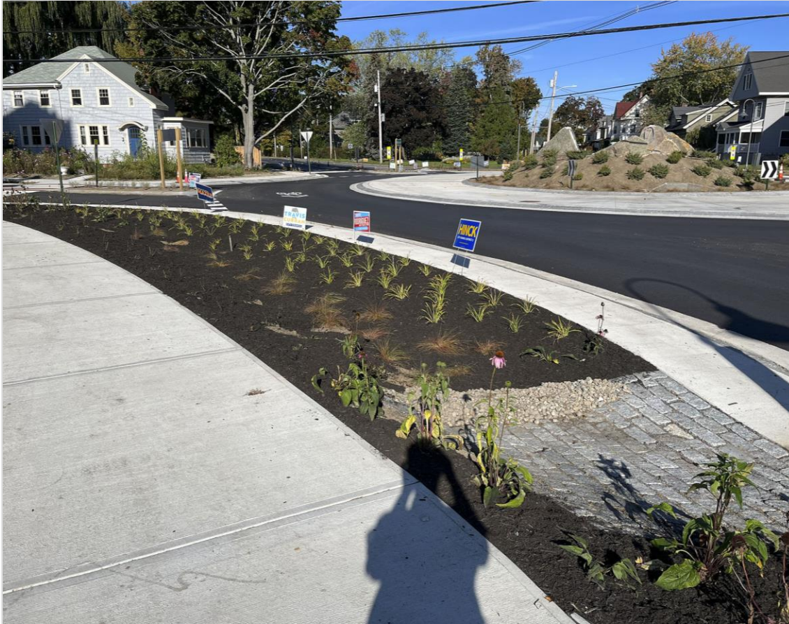
Deering Corner Roundabout Bio Retention Cells
